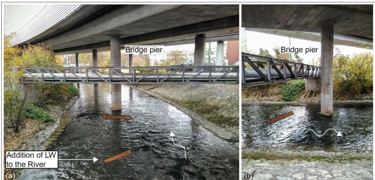
Figure 9. (a) Plan and (b) side view of the field test site at the River Glatt in Zurich (Switzerland) to study LW accumulation probability at a single bridge pier.
