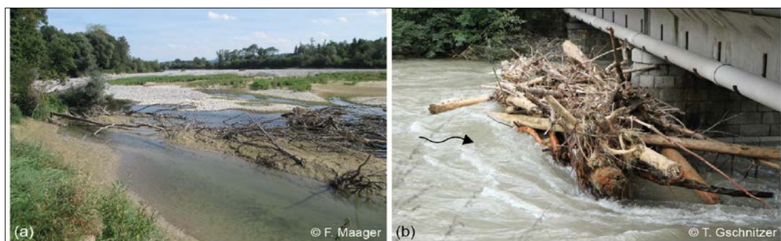
Figure 1. LW accumulation at (a) the River Thur, Switzerland, and (b) a bridge pier in Tyrol, Austria.
