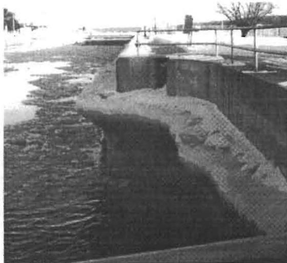
**Fig.5.** Ice collars in the gate recess and lock wall
