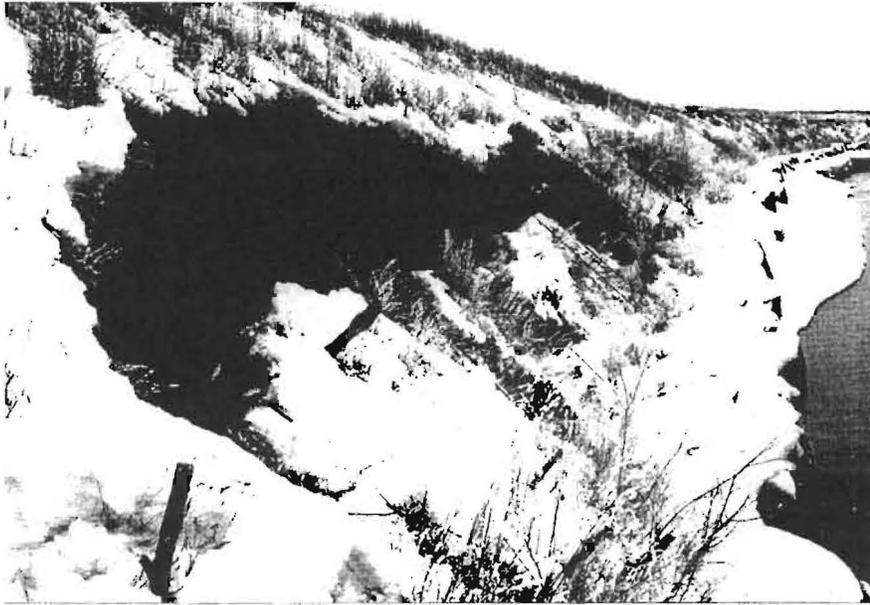
**Fig.3.** Bank failure consequent to ice-induced undermining of riprap
