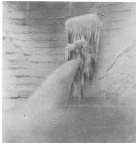
Figure 4. - View of ice accumulation on Morrow Point Dam outlet gate house due to spray and spillway gate leakage (spillway located above outlet works).
