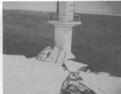
Fig. 4 Lake St. Peter-Breaking of ice floe by conical substructure
