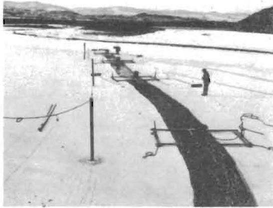
Figure 3. - View looking at channel cut in the ice at the Wind River Diversion Dam. Outboard motors are used to divert slush ice away from the power canal entrance .
