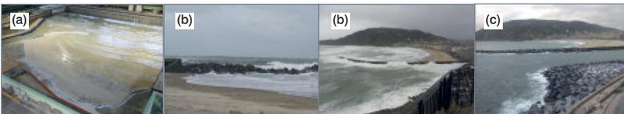
Figure 6. Zurriola beach. (a) Physical Model study (2013). (b) Damage in the 2013-2014 storms and (c) Situation in 2015 after repairs
