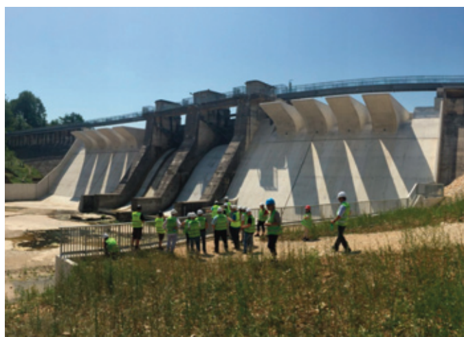
Figure 2. Charmines dam spillway in France with a 23 m wide type-A piano key weir section on both sides of the crest gates (PKW commissioned in 2015). Photo courtesy of EDF.
