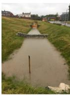
Figure 4: Swale under heavy rain conditions.
