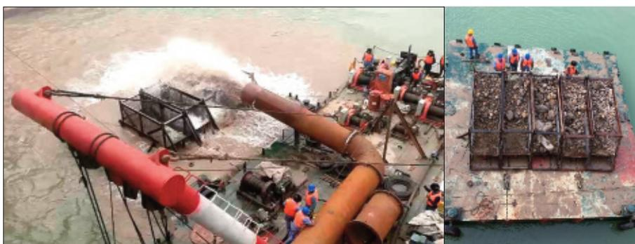
Figure 7. Dredging project of the tailrace canal of the Longkou reservoir in the Yellow River. The material diameter was 1 m.
