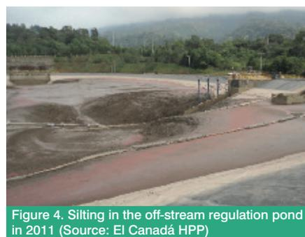
Figure 4. Silting in the off-stream regulation pond in 2011 (Source: El Canadá HPP)
