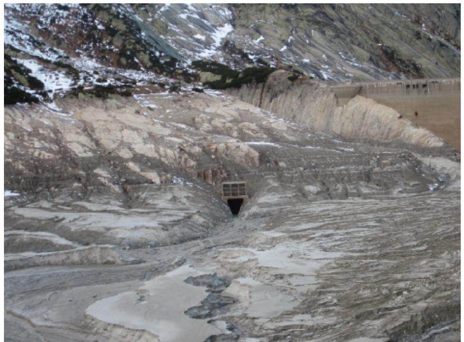
Figure 1. Räterichsboden reservoir in Switzerland during the emptying operation in 2014. The view is toward the bottom outlet (center) situated right below the power intake. Carved channels with steep-sloped banks on the sediment deposits converge to the bottom outlet. The dam and spillway are on the background on the right-hand side. Photo: M. Müller
