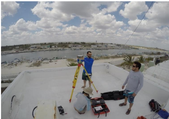
Figure 8: GPS base-unit installation
