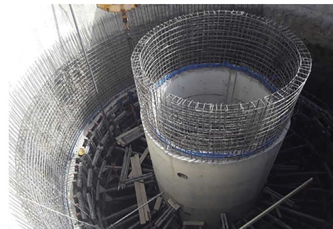
Figure 5 | A 4 m -diameter drainage well of the Hay Sadri neighborhood stormwater tunnel, part of the SRE system in eastern Casablanca.
