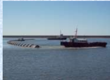
Installation of Mar del Plata outfall
