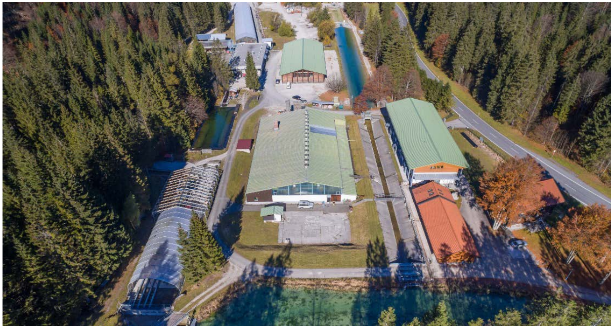
Figure 2: Oskar-von-Miller Research Institute for Hydraulic Engineering in Obernach, Germany (TUM)
