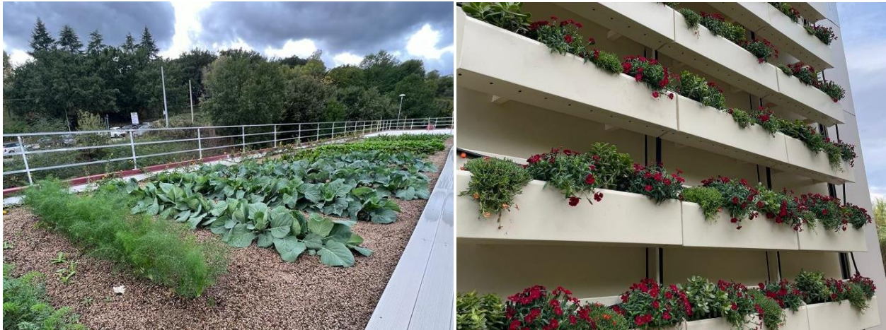
One of the two innovative green roofs (the agricultural one) on the left side and the green wall system on the right side. The pictures were taken by the research team of the LIU.
