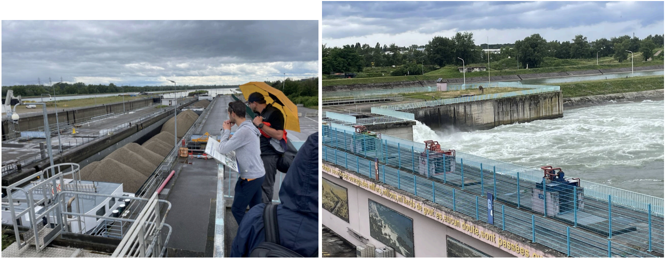
EDF guided visit - the lock and the dam
