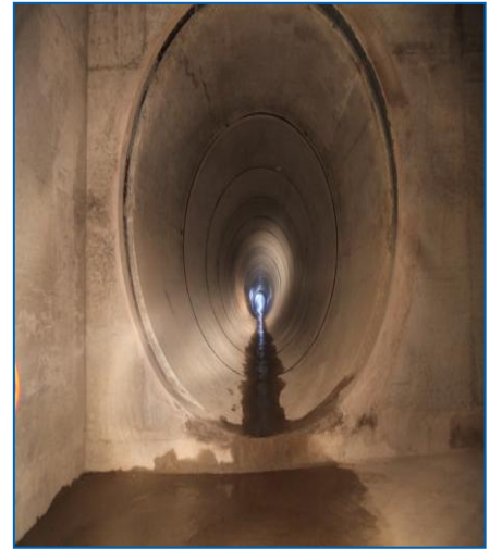
Interior of Wuluju Double Pipelines (3m in diameter)
